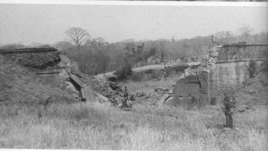
Going . . . going . . . gone . . . One of the bridges destroyed in Mozambique
